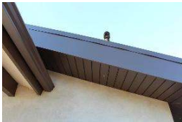
Steel Fascia Board
